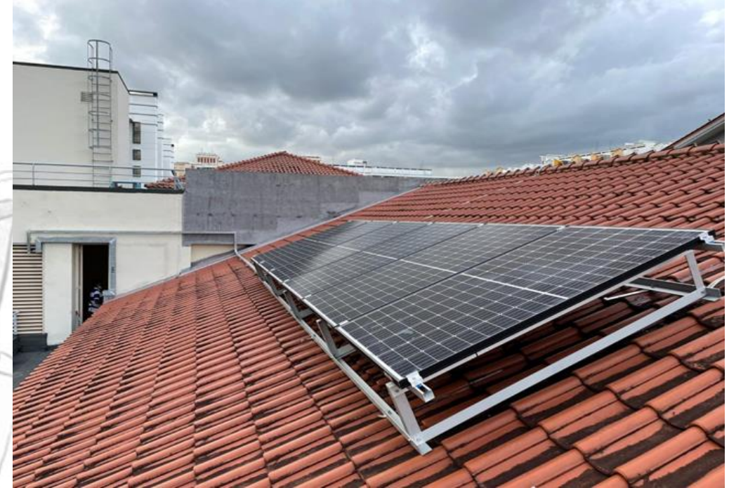
Latest installation of hybrid solar panels (Dec 2020)
